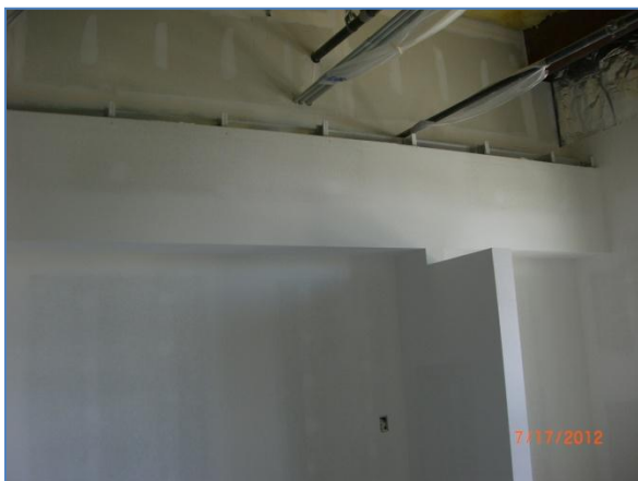
Soffit framing at third floor
