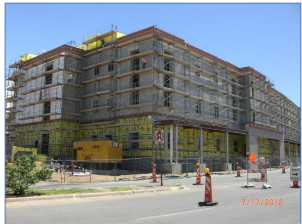
Exterior building looking southeast
