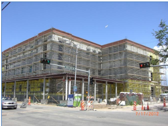
Exterior building looking northeast
