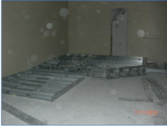
Framing raised platforms at courtrooms
