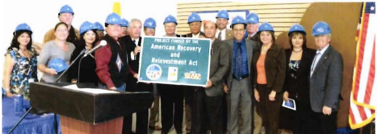
Marking the start of construction on NCRTD's facility in Espanola, NM, are, from left: front row, Mary Lou Quintana, Santa Clara Pueblo; Jennifer Catechis, representing Rep. Ben Ray Lujan (D-NM); Michele Jacques-Ortiz, representing Sen. Tom Udall (D-NM); Elias Coriz, Rio Arriba County commissioner; Jack Valencia and Ivan Guillen of NCRTD; Alfred Herrera, chairman of the NCRTD board; New Mexico DOT Adjutant Secretary Rebecca Montoya; Josette Lucero, NCRTD executive
