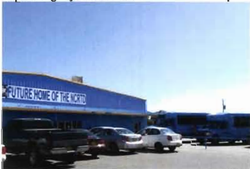
Future Home of the NCRTD – The Jim West Regional Transit Center, Espanola, NM
