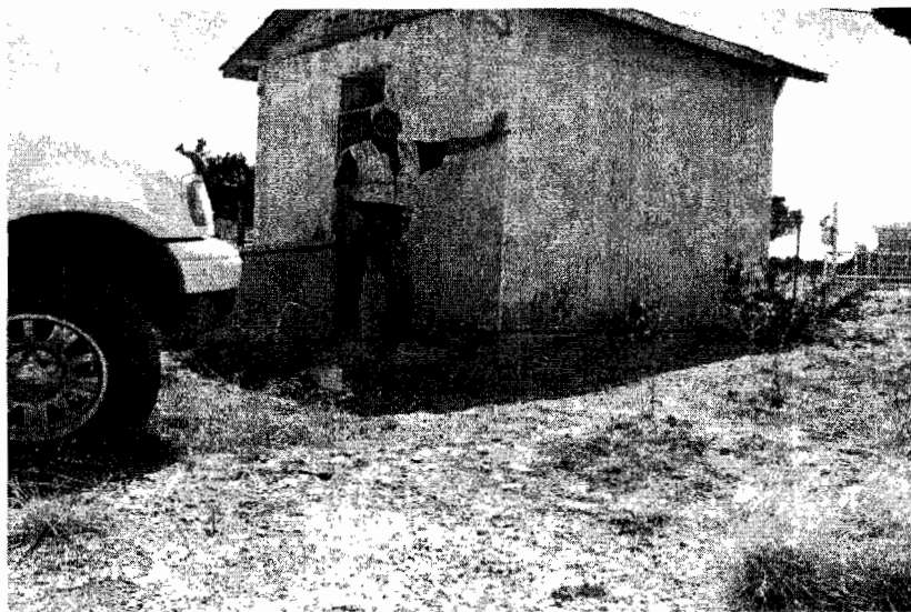
Exhibit B. Well house and well (Owner Tom George in picture)
