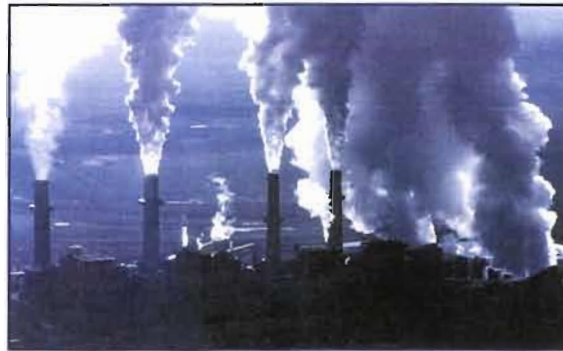
Four-Corners power plant
