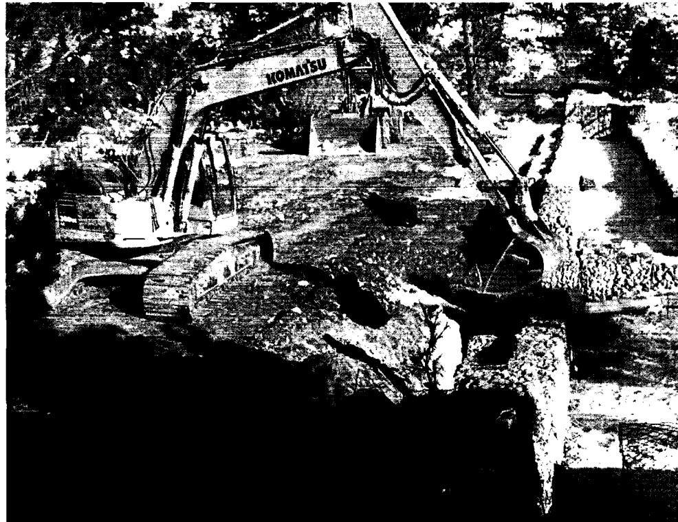
Building the structure across Pueblo Canyon
