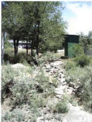
A cobble-lined swale emptying onto Cave Road
