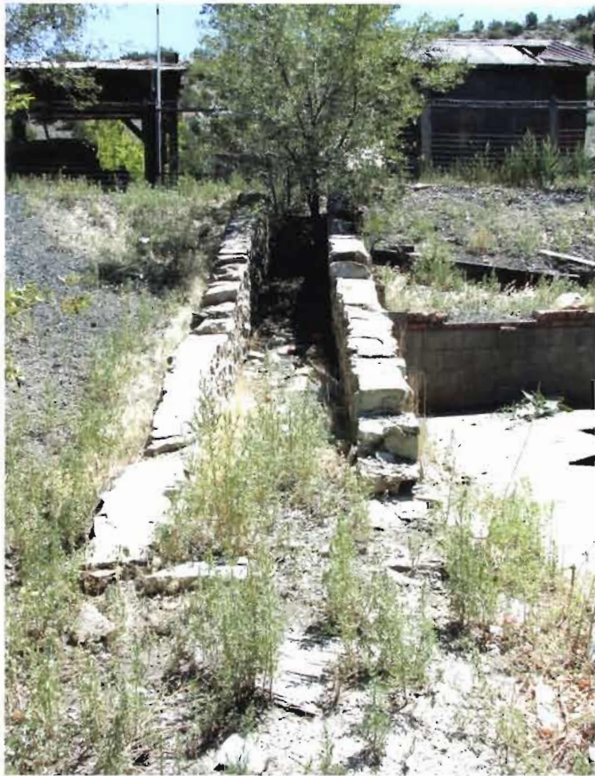
Stone drainage flume on Main Street - an example of vernacular design
