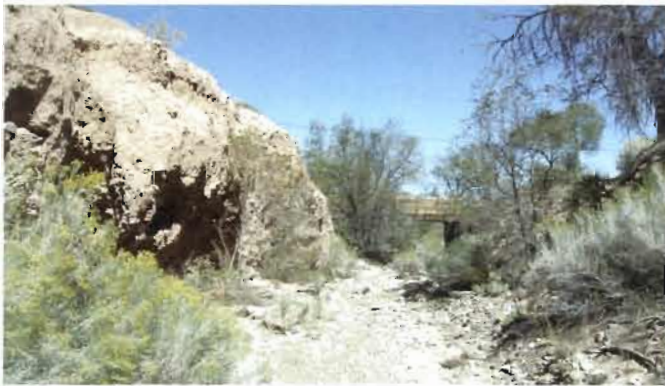
Pedestrian bridge, beyond, and arroyo escarpment. This portion of the Madrid arroyo was channelized and straightened in the 1930's by the US Army Corp of Engineers.
