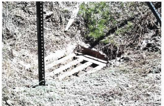
Existing drop inlet on the east side of NM 14.
