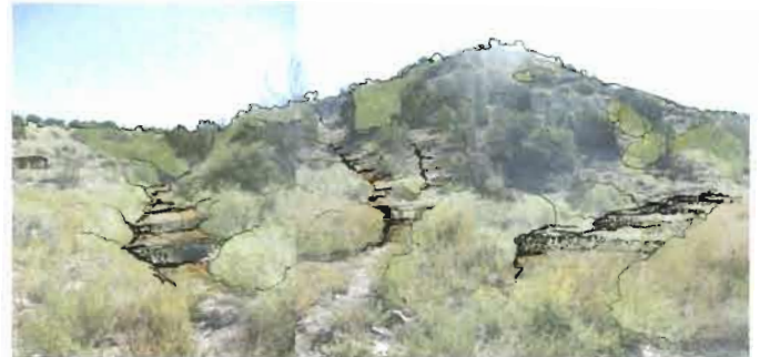
Potential gabions, stone check dams, one-rock dams and stabilization on the east slope
