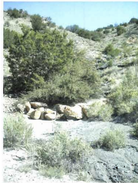
Stone grade break in arroyo behind the Mineshaft Tavern, an AML sponsored project.
