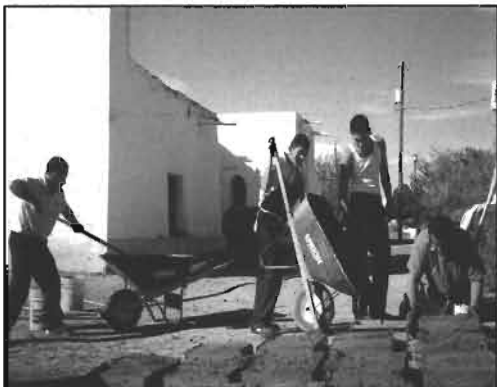
Socorro, TX—Youth training, making adobe
