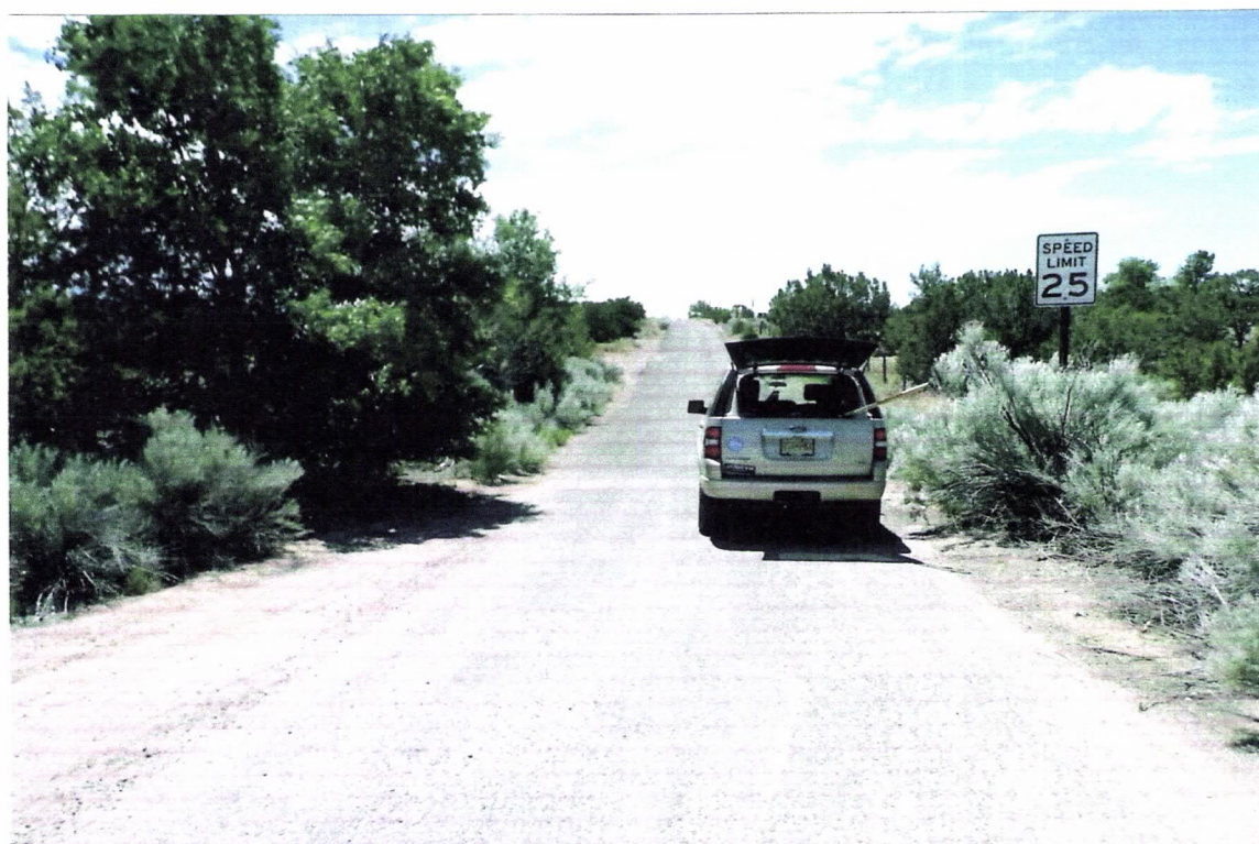
Camino Peralta 3 feet south of Camino Espejo intersection showing car in roadway, looking south. Road is 13 feet wide.
