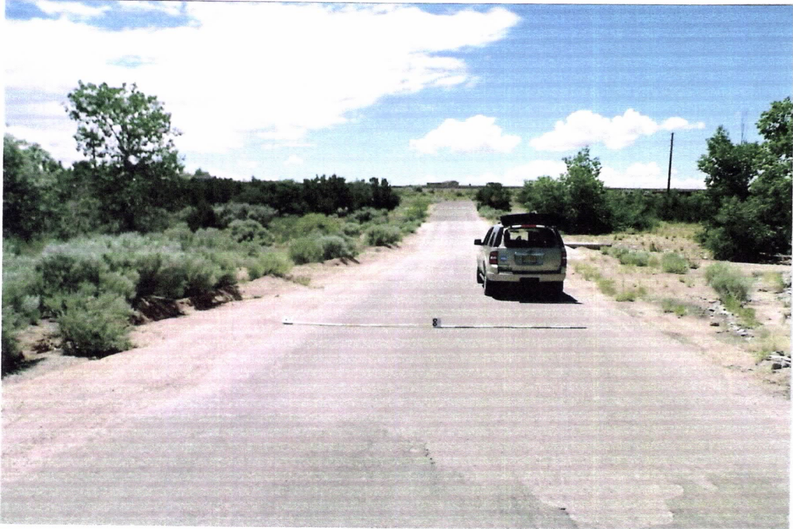
Entrada looking south toward entrance to Puesta del Sol showing concrete pad crossing Las Trampas arroyo, showing car in roadway. Road is 17 feet wide.
