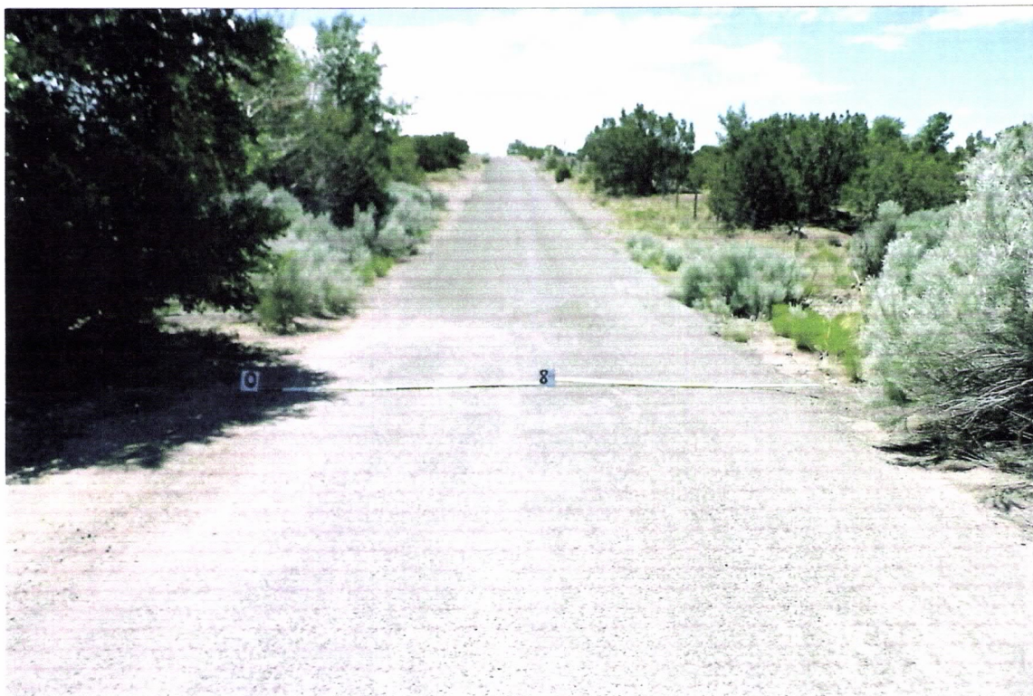
Camino Peralta 3 feet south of Camino Espejo intersection, looking south. Road is 13 feet wide.
