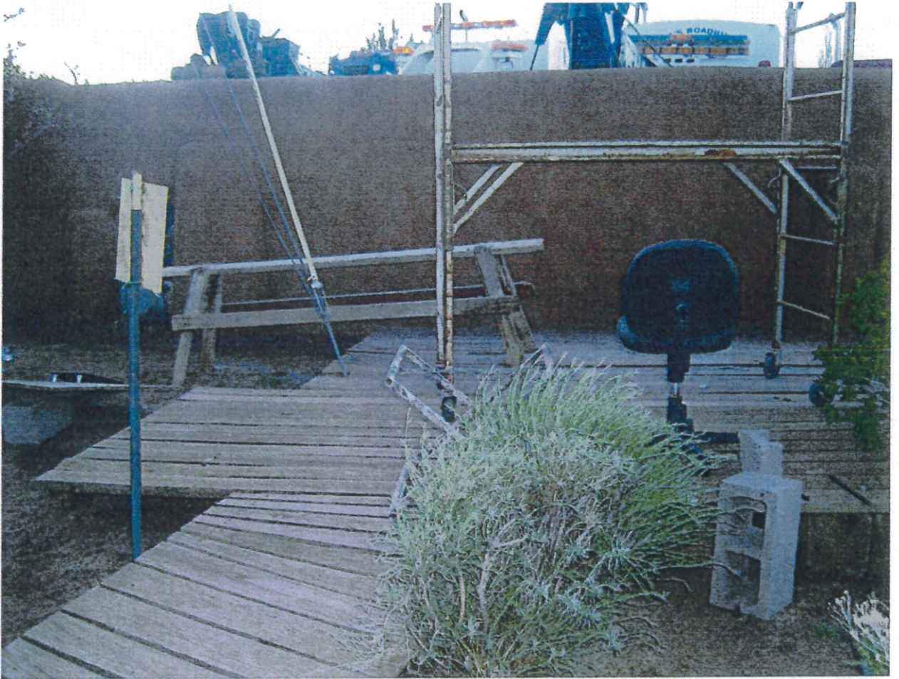
PICTURE 12: DAY THE REPAIR ON THE WALL WAS COMPLETED
