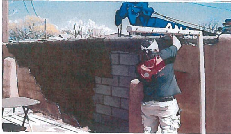
Picture 10, 11: Anaya refused to move his trucks while wall was being repaired or allow workers to go on his property though there was a Mutual Restraining Order in place.
