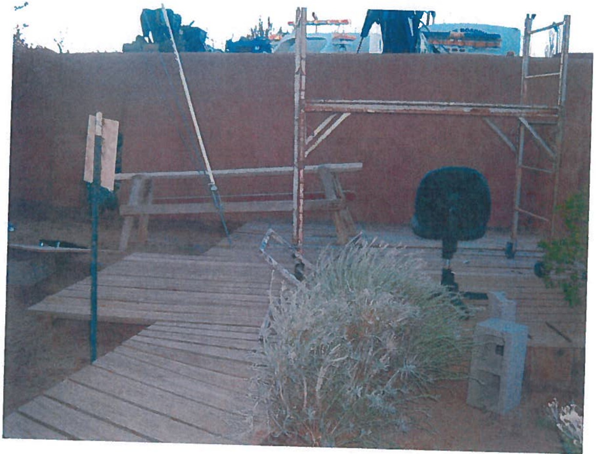
PICTURE 12: DAY THE REPAIR ON THE WALL WAS COMPLETED
