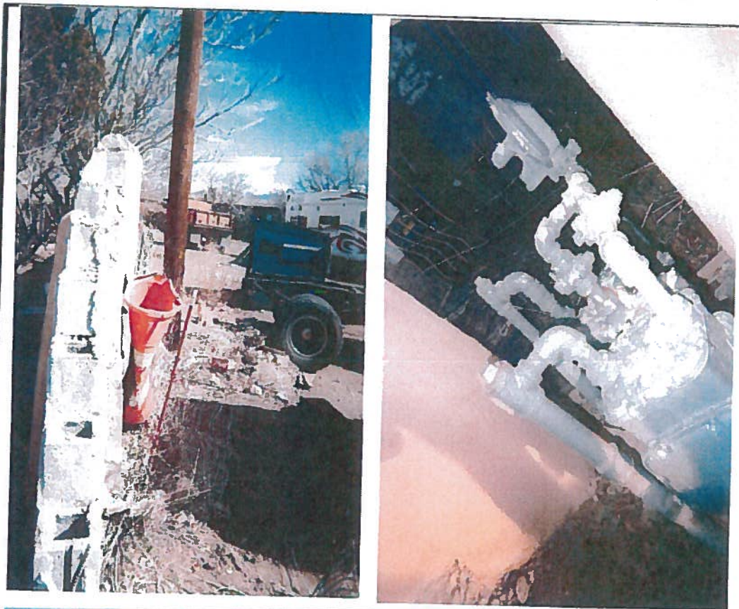
Picture 4, 5, 6, 7, 8, 9, 10, 11: (3 Pages) Anaya yard from January 14, 2012 to March 27, 2012 showing yard condition and trucks backed into wall, fence, gas meters and temporary privacy pellets.
