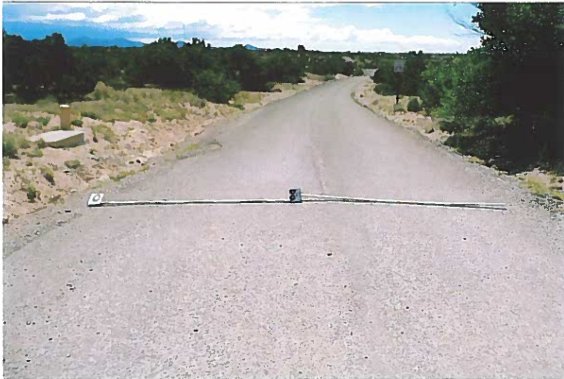
Camino Peralta at top of rise between Terra Bella gate and Camino Espejo, looking south. Road is 17 feet wide.
