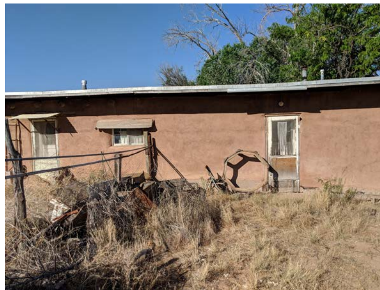
Montoya Adobe home
