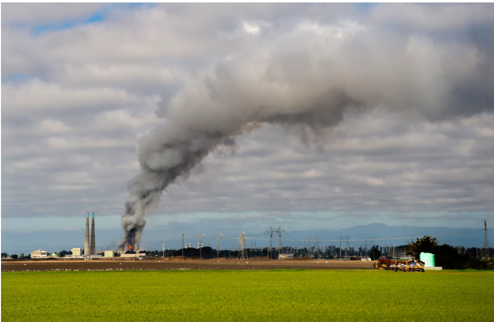
Smoke and flames are seen from Castroville as a fire at the Vistra battery storage plant burns in Moss Landing, Calif., on Friday, Jan. 17, 2025. Less than two weeks after the fire, scientists affiliated with San Jose State University discovered levels of toxic metals at more than 100 times the normal
