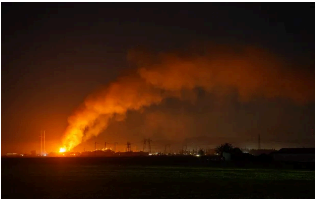
Smoke and flames are seen from Castroville as a fire at the Vistra battery storage plant burns in Moss Landing, Calif., on Thursday, Jan. 16, 2025. (Doug Duran/Bay Area News Group)
