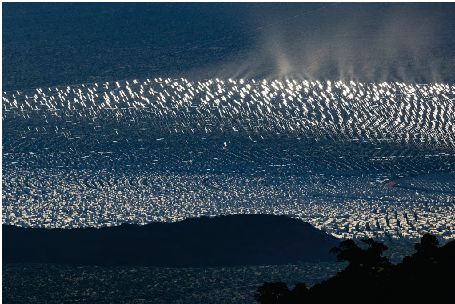
Mirrors sprawl across the desert at the Ivanpah solar electric generating system near Nipton, California. Photograph: David McNew/Getty Images
