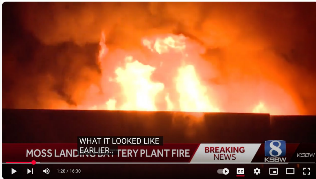
Moss Landing battery plant fire update at 11 p.m. 1/16/25
