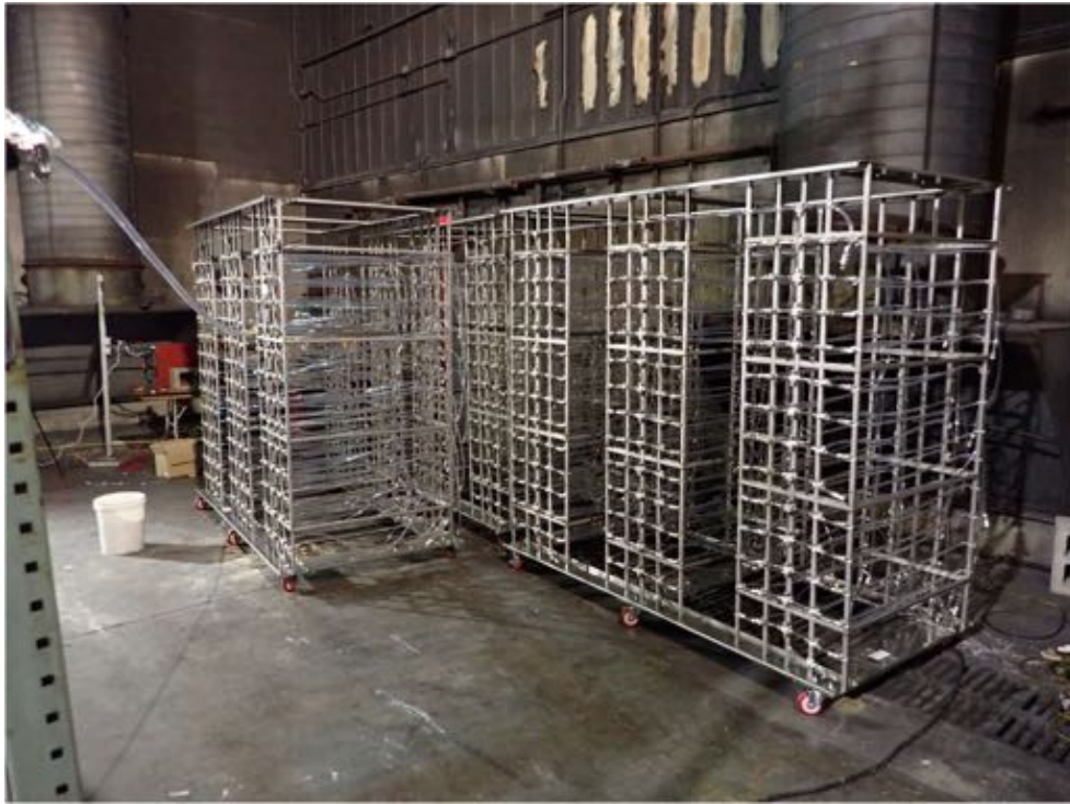
Figure B7 – Dummy Racks with NOVEC Piping 6
