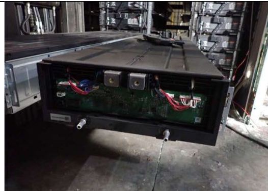
Post Test – Front View of Module 9
