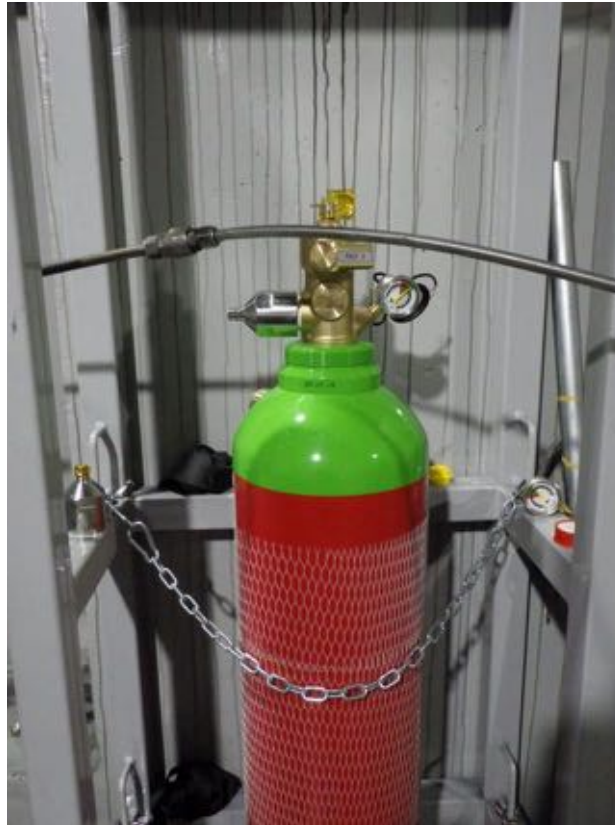
Figure F2 – Photo of Novec 1230 Cylinder
