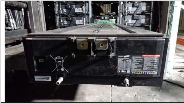
Post Test – Front View of Module 11
