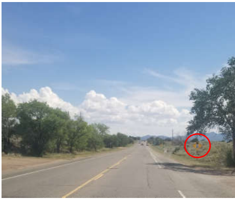
Figure 6: NM 14 Southbound Reduce Speed Limit Ahead Sign
