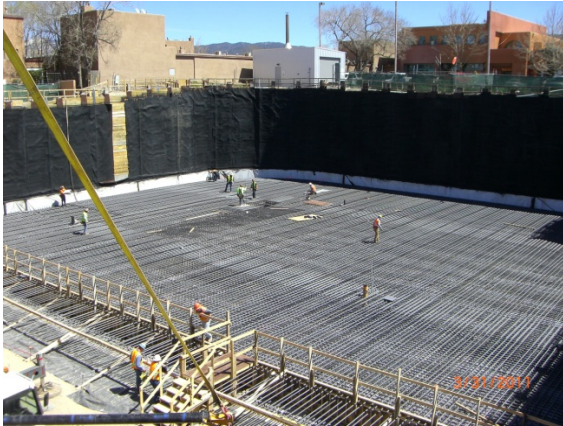
Upper mat rebar placement at east half of lower basement
