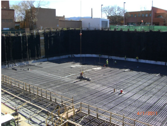
Rebar dowels for walls started at east half of lower basement
