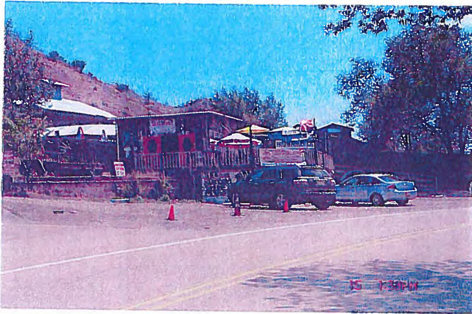
Madrid Historic District old coal mine shaft museum along NM HWY 14.
